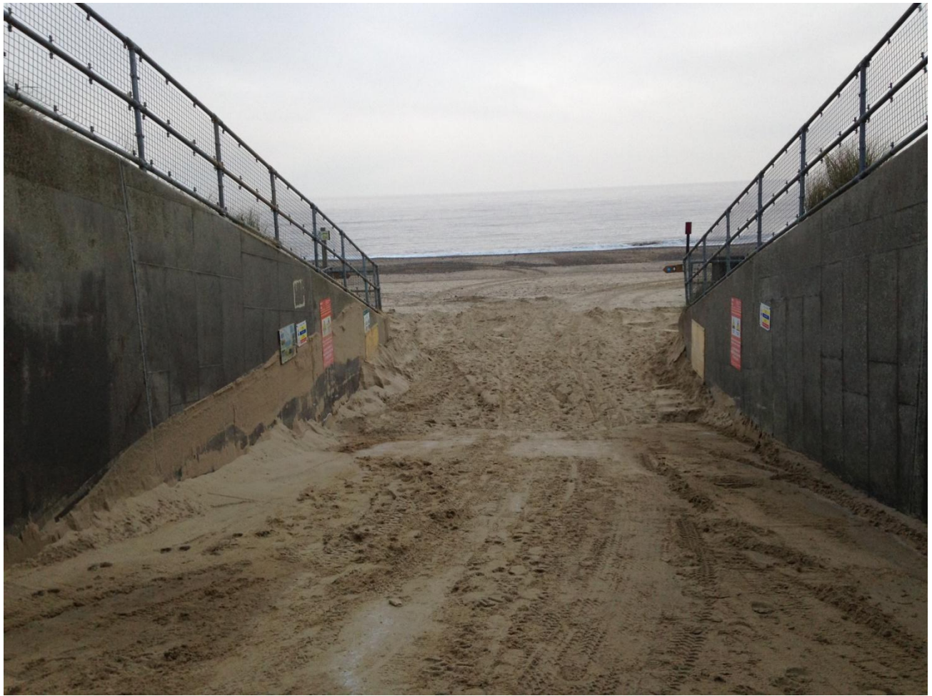
Figure 38. Site 4a. Beach access at North Gap. HDD alignment is 70m to the right of the photograph.
