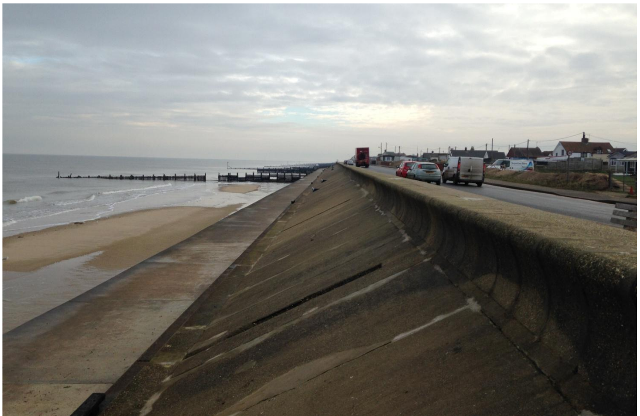
Figure 29. Site 1. View to Southeast from above the potential HDD alignment showing coastal defences and B1159.
