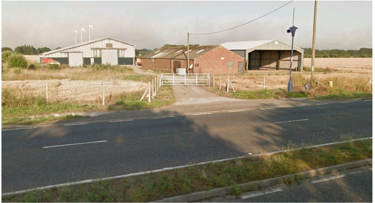
Figure 46. Site 8. Google Street View Photograph of potential access point from the A12. HDD entry point is beyond the line of the trees in the distance.
