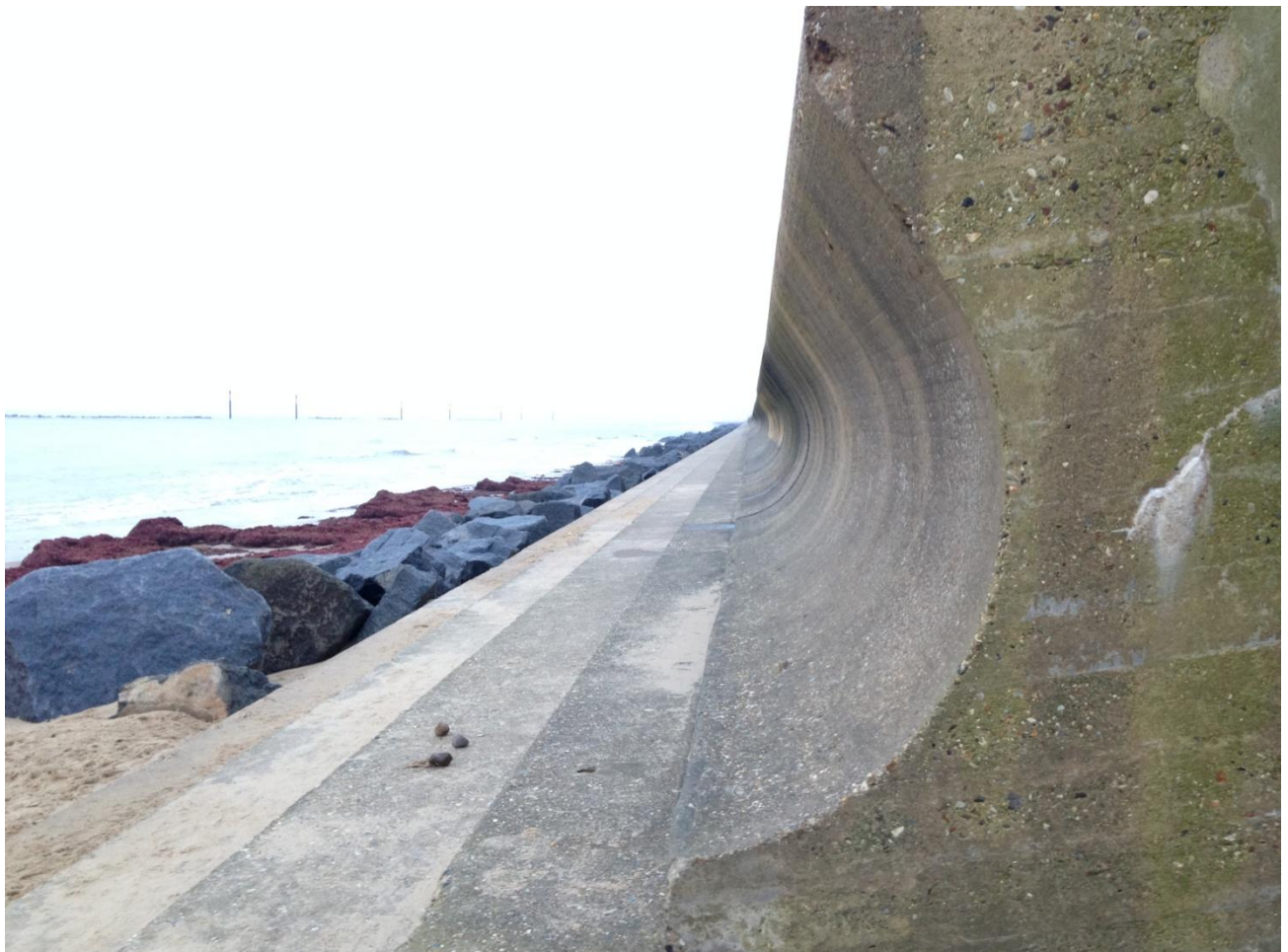
Figure 41. Site 5. Beach defences looking south east from Sea Palling beach access. Offshore rock walls are 250m from the shore. The concrete shoreline defences continue beyond the HDD alignment, 300m from the viewpoint. Alignment 5 passes to the left of the offshore rock wall on the left of the photograph.
