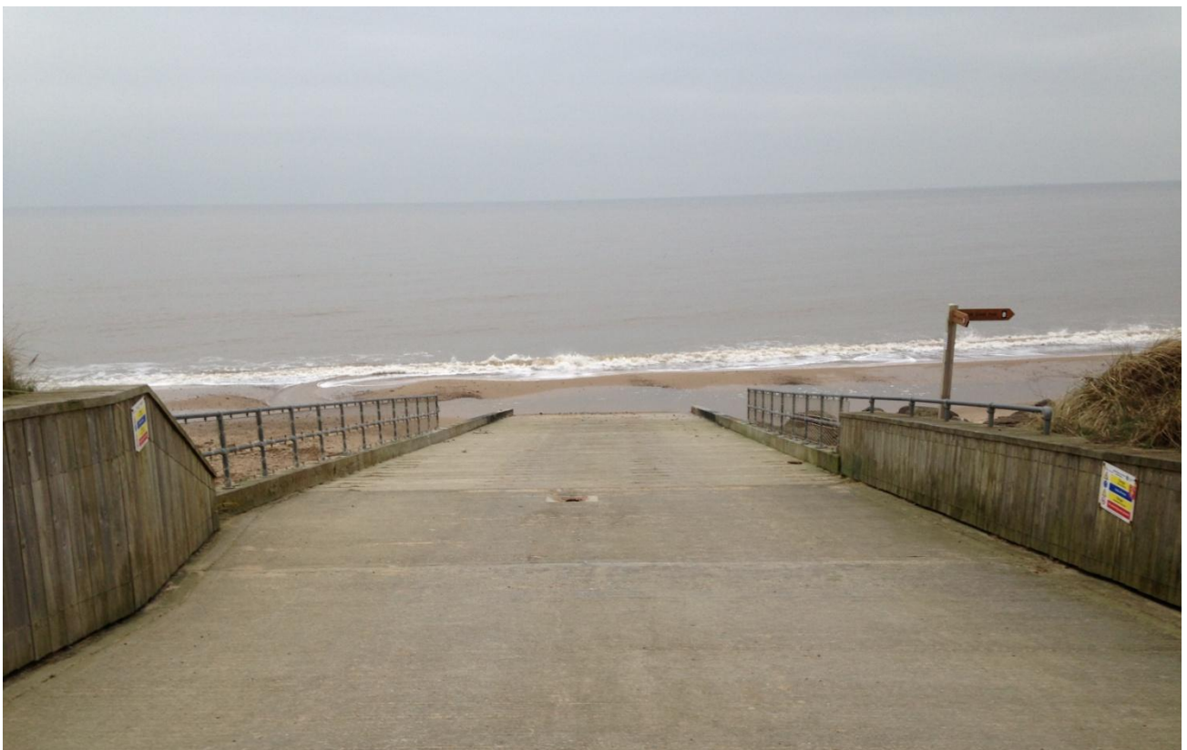
Figure 35. Site 3b. Beach access ramp at Cart Gap, adjacent to Site 3b.
