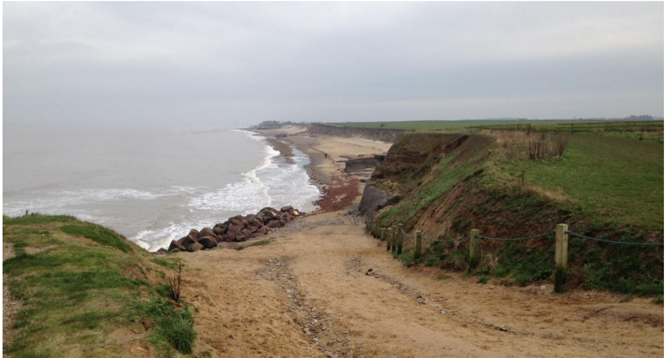
Figure 32. Site 3a. View to southwest from beach access. Beach access will periodically require reinstatement as coastal erosion advances. Site 3a entry point is in far distance before the small headland.
