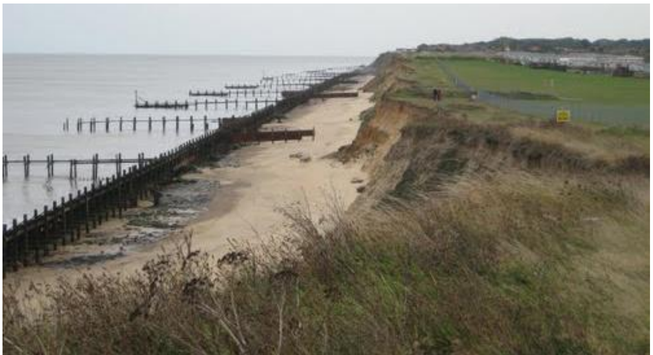
Figure 51. Site 9. Google Earth Panoramio photograph viewed southwards towards Broadlands Sands Holiday Park. Site 9 HDD route crosses the cliffs 50m beyond the people in mid distance. Erosion has since reached the boundary fence, taking the coastal footpath and preventing access. Vehicle access to a short HDD exit position would be very difficult due to sea defences.
