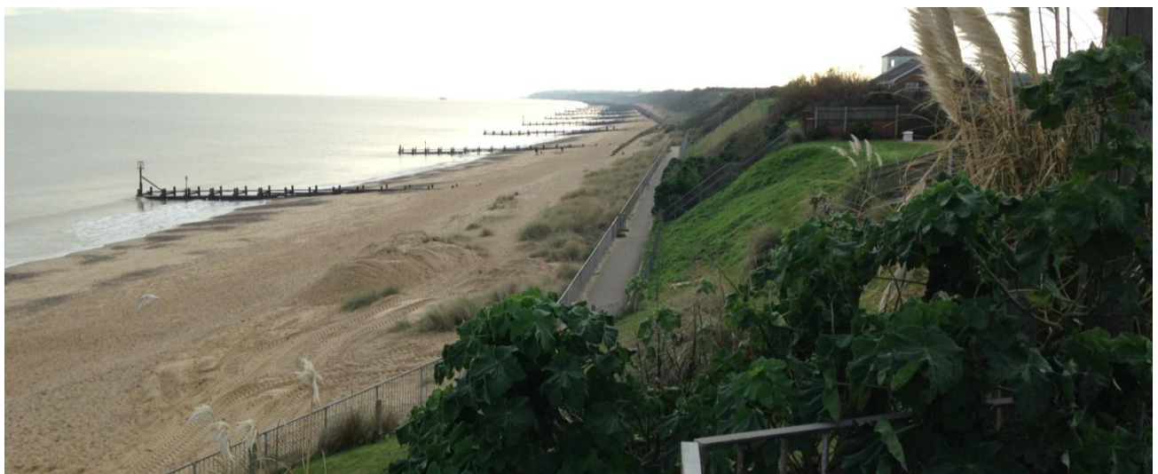
Figure 49. Site 8. View southwards towards Site 8 from Marine parade Gorleston. Site 8 HDD alignment is located at the 5 th Groyne along.
