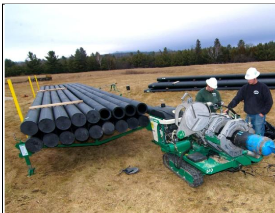
Figure 18. Typical setup of PE butt fusion welder
