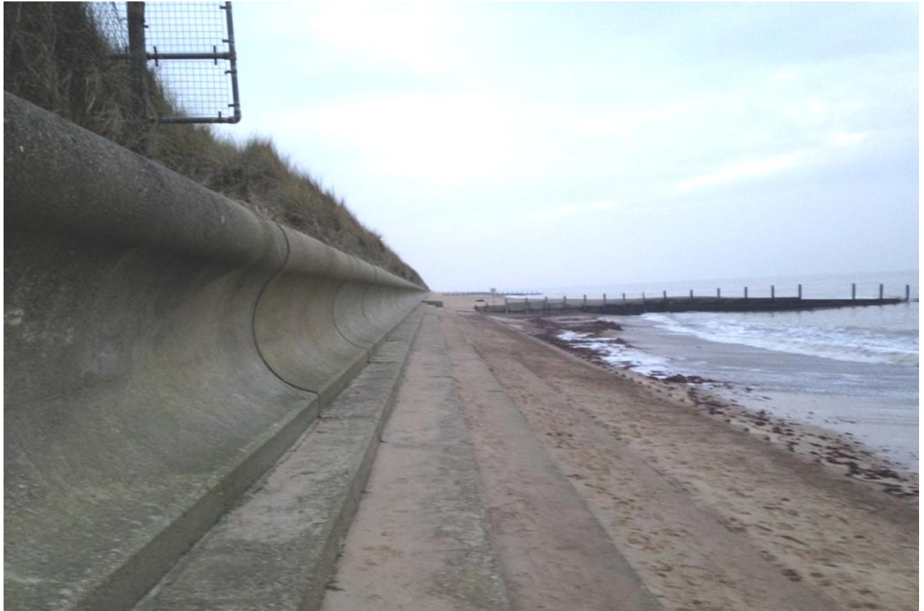
Figure 44. Site 7. Sea defences at Site 7 looking to the northwest.
