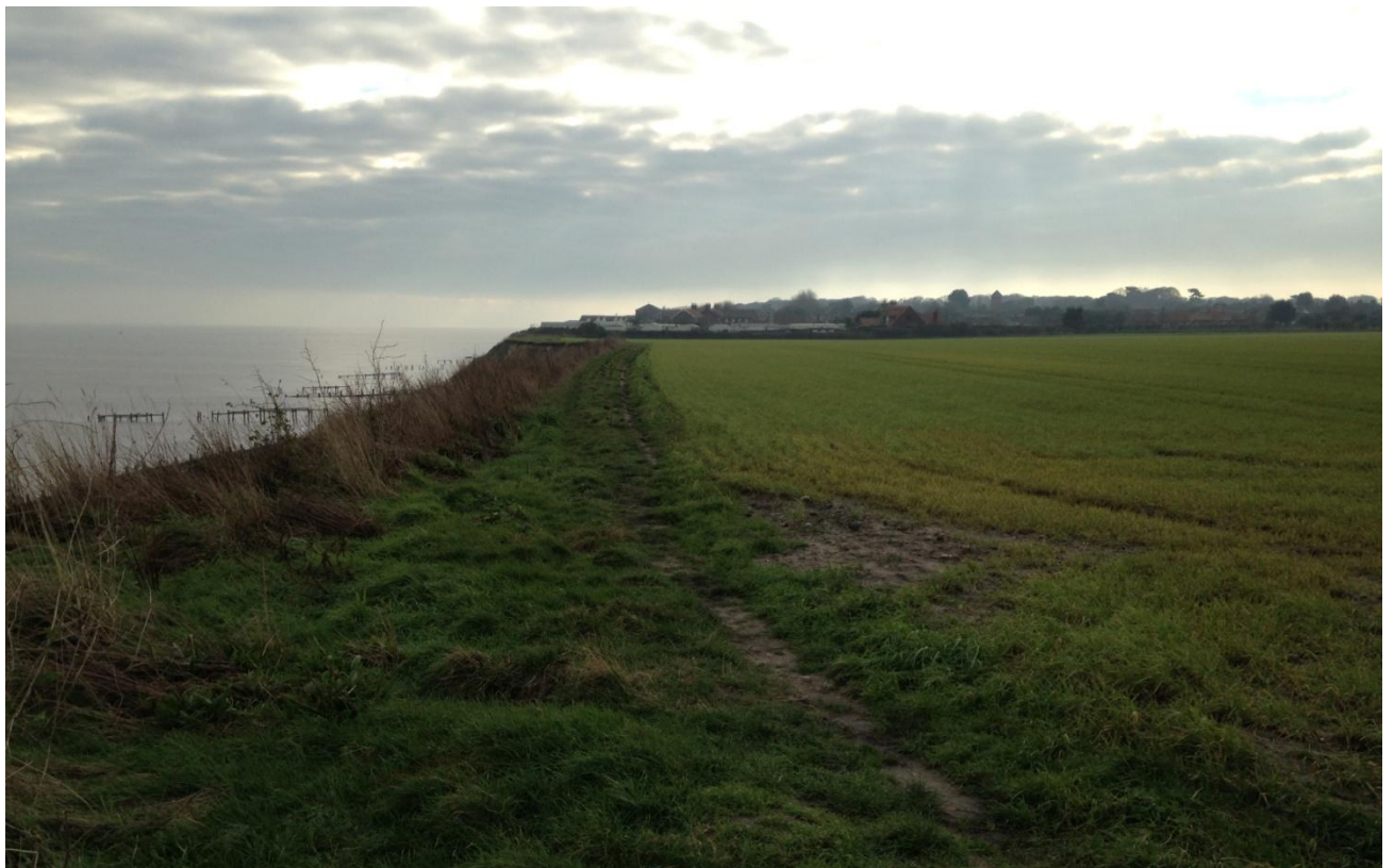
Figure 53. Site 10. View southwards towards the route of Site 10 HDD, approximately in the middle of the field. Coastal defence structures can be glimpsed on the left of shot.
