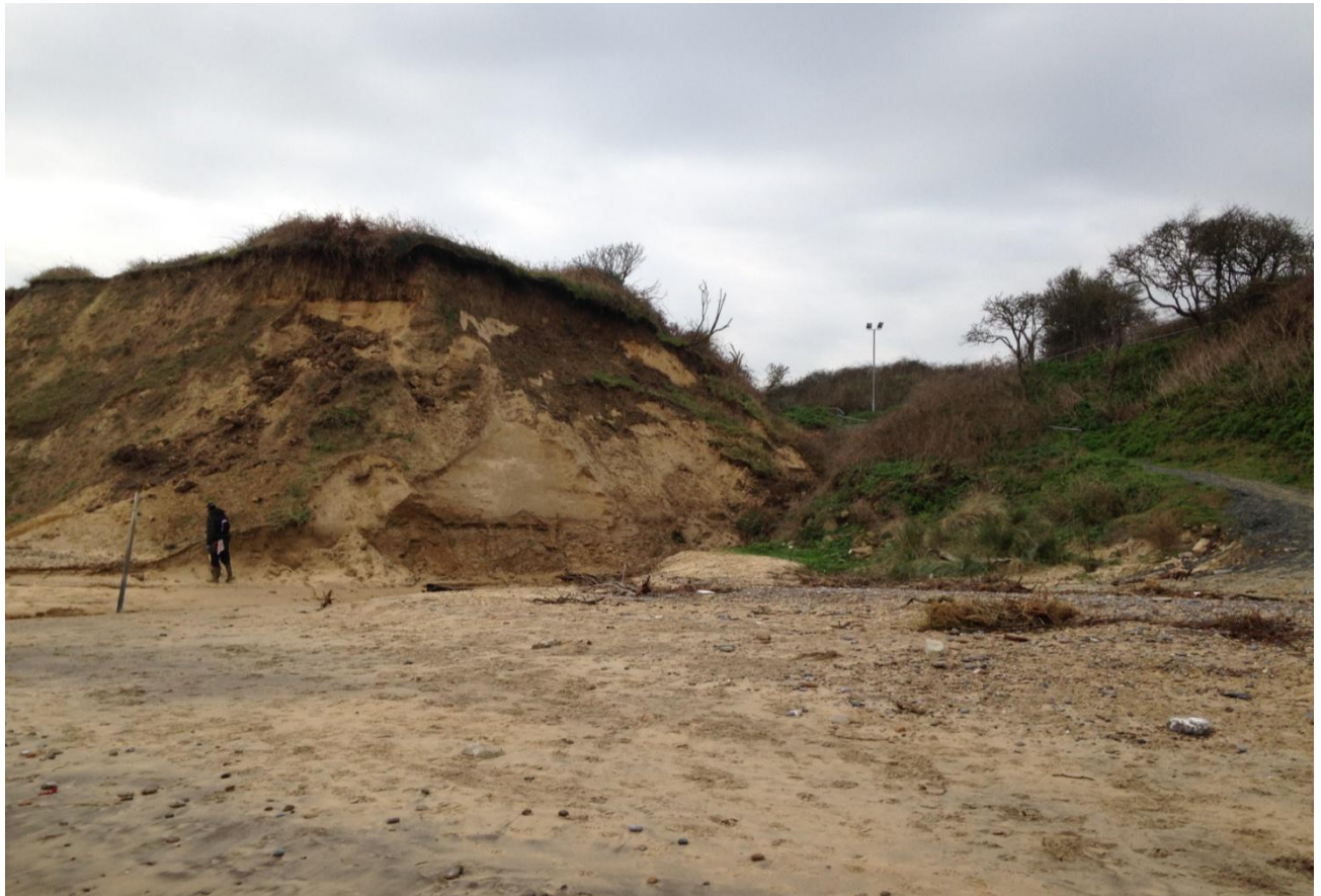
Figure 59. Site 12. Footpath to Pakefield Coastwatch Tower showing eroding cliffs of fine sand.
