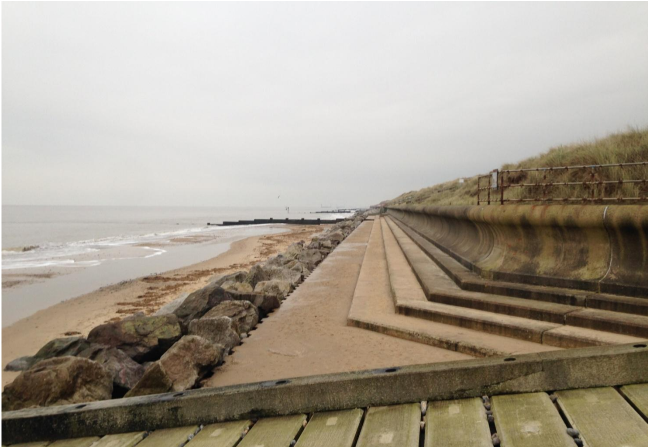
Figure 36. Site 3b. View south from beach access ramp. HDD alignment will be between the ramp and the wooden groyne in mid distance.
